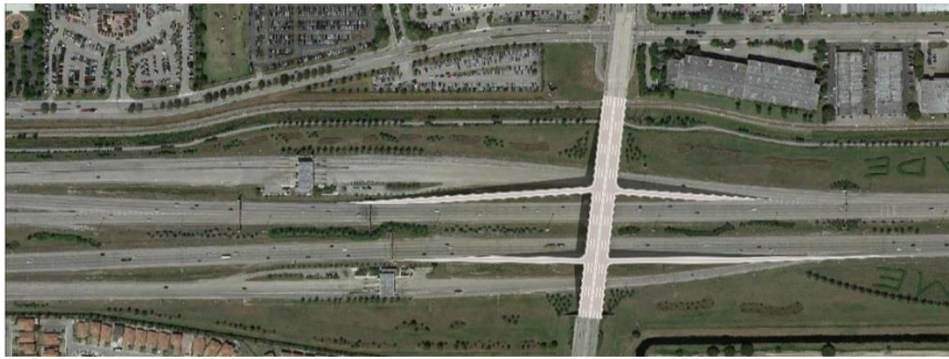
Figure 19: SR 836 On-Off Ramp at NW 97th Avenue
